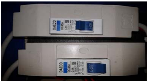
Gambar 19. MCB ( Miniature Circuit Breaker )
